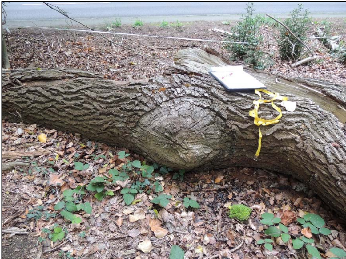
Photo 1: Tree inspectors should be particularly cautious when assessing the potential for failure associated with large occluded wounds on mature trees, especially when associated with other factors such as poor health or additional structural defects.
